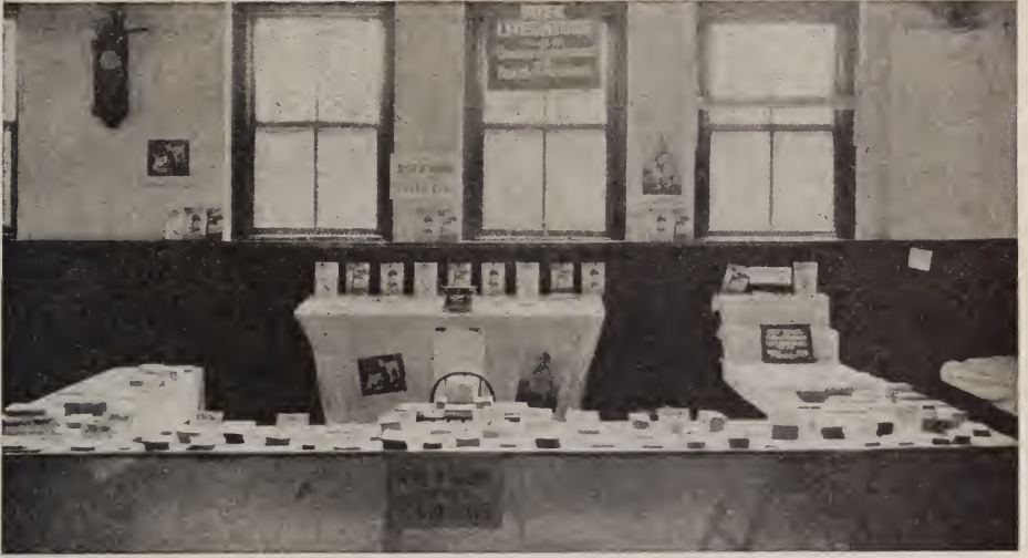
IN THE BASEMENT AT TEMPLE BETH EL
